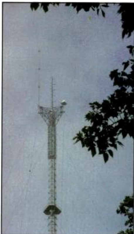
A candelabra on the top of the WBNS tower (Columbus, OH) holds the WBNS-TV and WCMH-TV antennas and an ENG receive site. A multistation FM panel antenna is mounted just below the candelabra.
